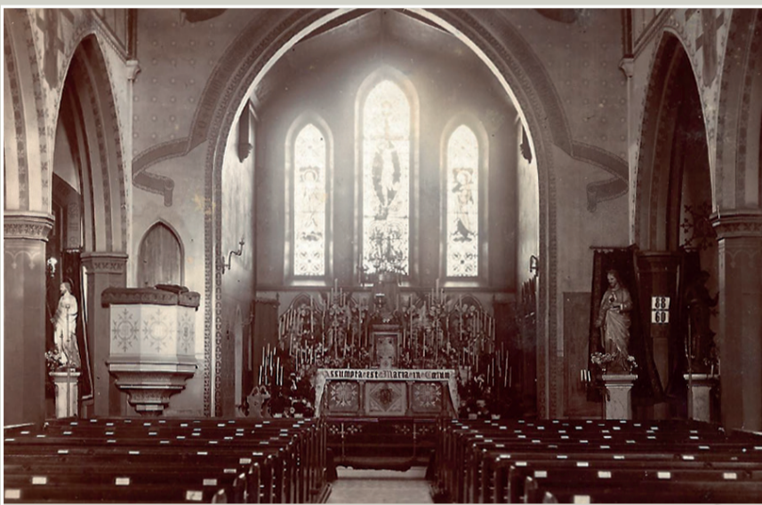
Early twentieth century photograph of east end (Diocesan archive)
